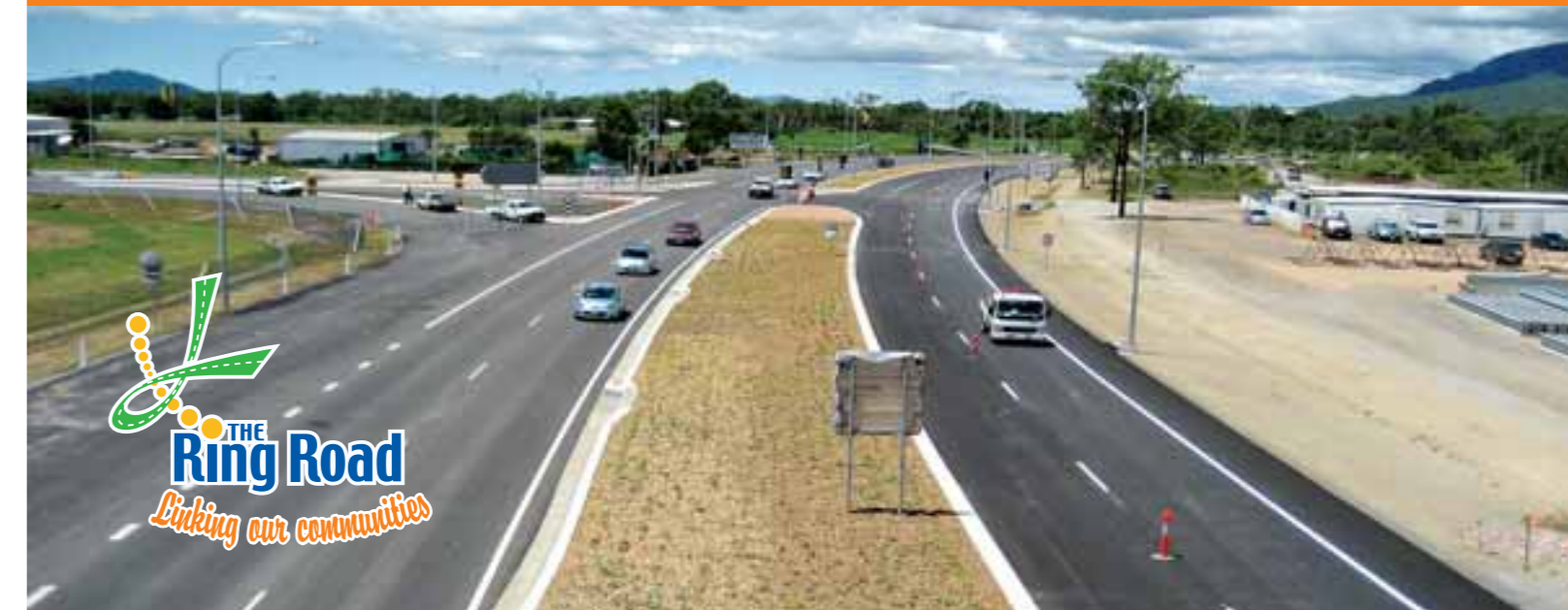
Looking east from the Ring Road's Hervey Range Road overpass to the on and off ramps for the Ring Road (left) and the project site office (right).
