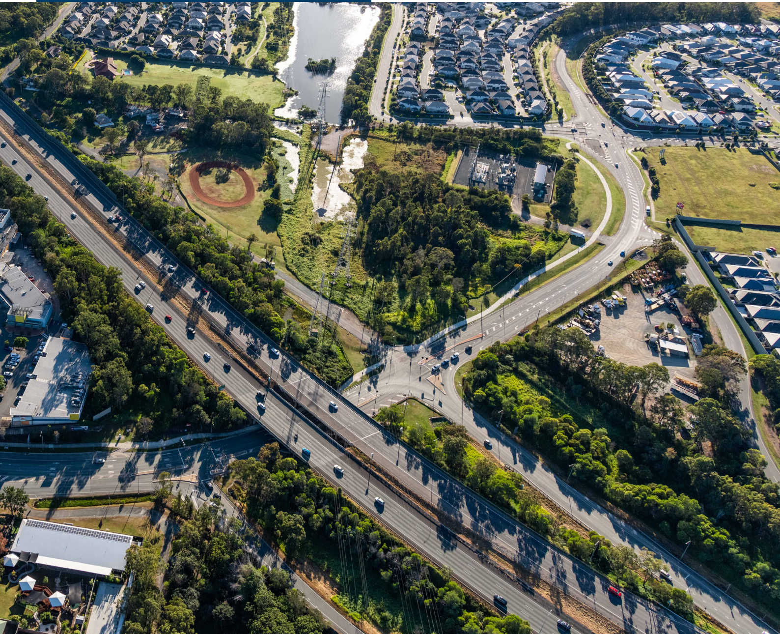
Bruce Highway at Dohles Rocks Road Interchange. Source: TMR
