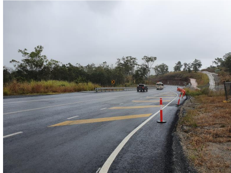
Figure 3: Northbound traffic on the MC001 alignment completed in 2019
