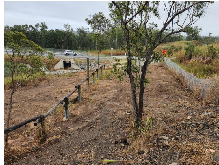
Figure 5: Koala sensitive infrastructure prior to landscaping activities
