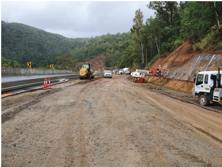
Figure 4: Pavement and shotcrete works at upper hairpin
