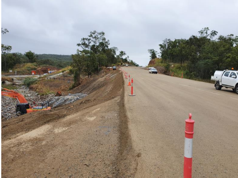
Figure 2: New MC002 (southbound) alignment under construction
