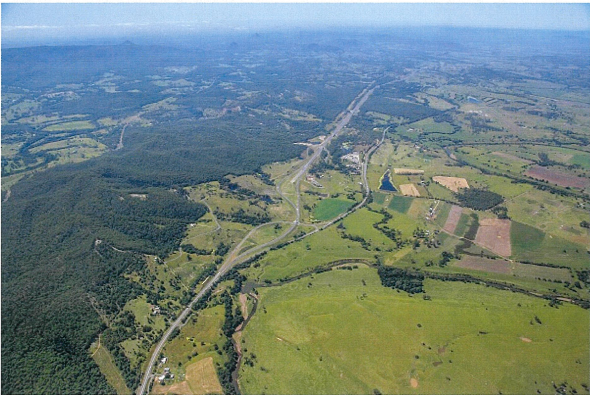
Figure 3 Completed Highway - Looking north to Woondum Interchange
