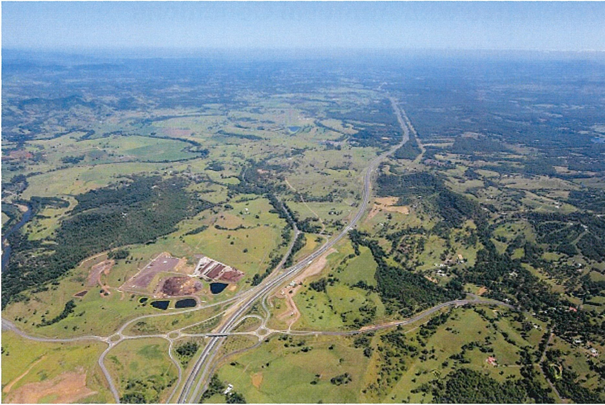
Figure 2 Completed Highway - Traveston Interchange north to Woondum
