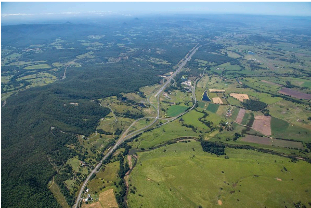
Figure 3 Completed Highway - Looking north to Woondum Interchange
