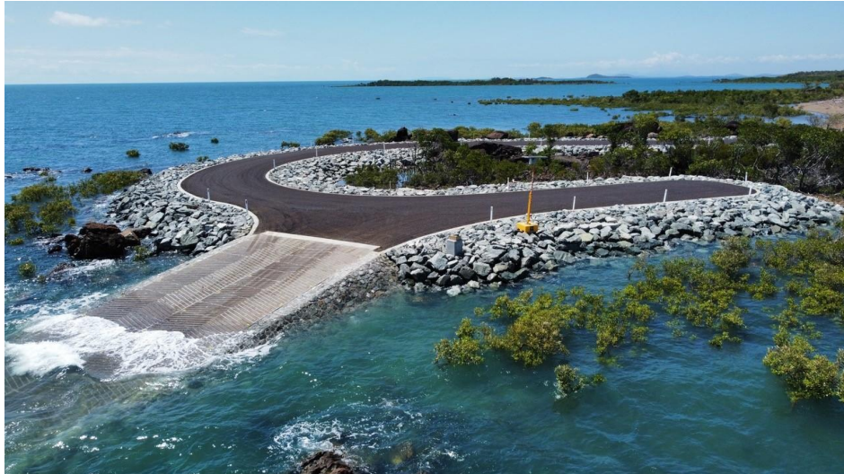
Caption 7: Midge Point (Queensland) boat ramp.
