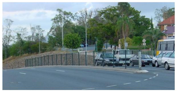
Figure 1.1-A – Fences can be installed on medians to control pedestrian movements
