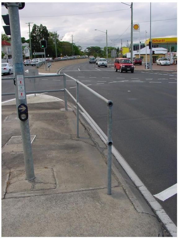
Figure 1.1-D – Fencing and barriers constructed using a horizontal rail should not be used because of the risk of spearing pedestrians and vehicle occupants during a crash
