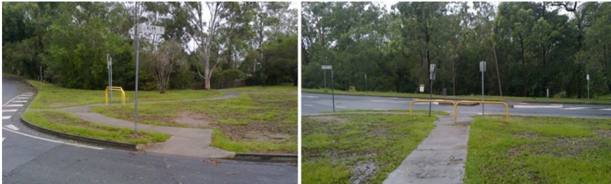
Figure C.4 – Redundant U-rail type terminal barrier
