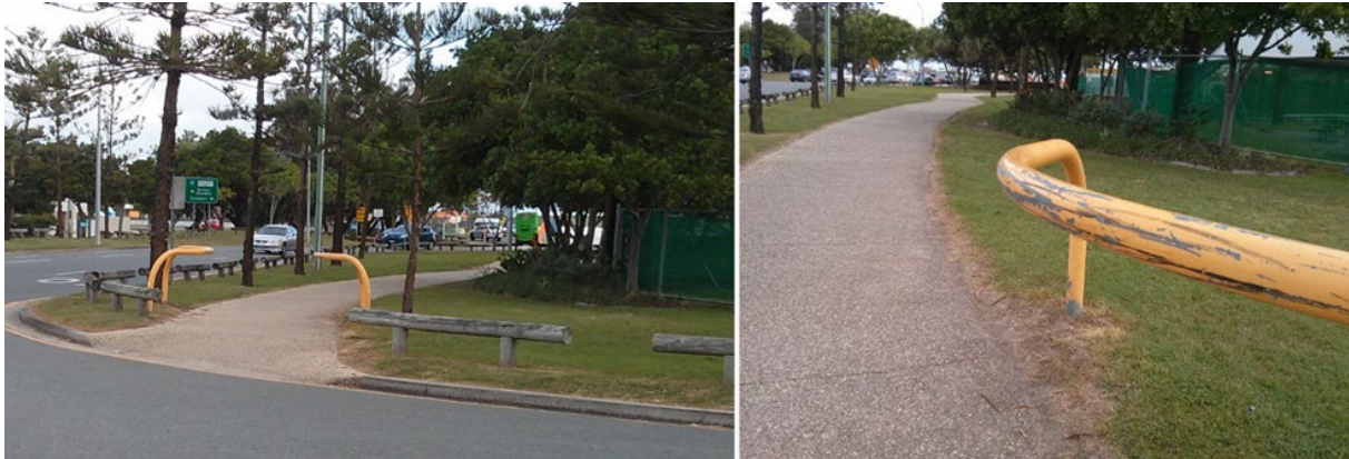
Figure C.16 – Damage which indicates evidence of insufficient passing width
