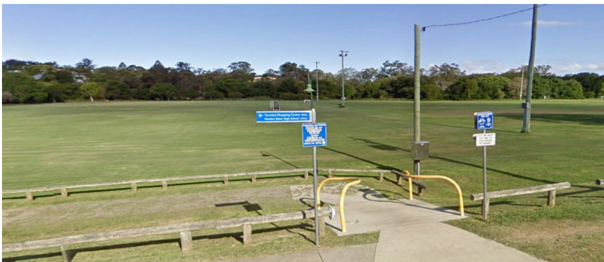
Figure C.6 – Hazardous positioning of a path terminal barrier
