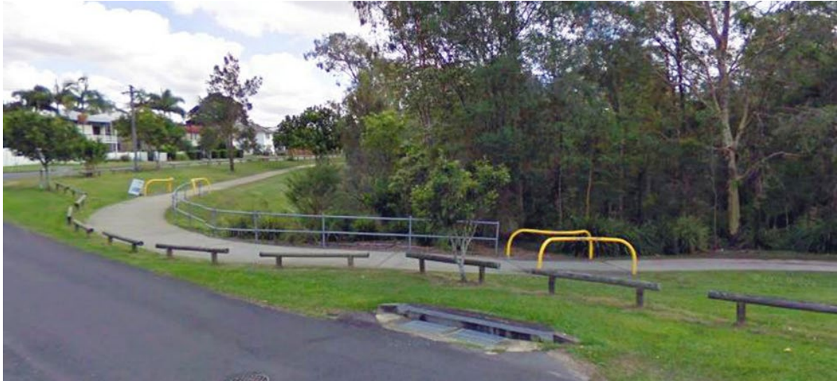
Figure C.2 – Excessive use of physical barriers to slow people riding bikes on approach to a blind corner
