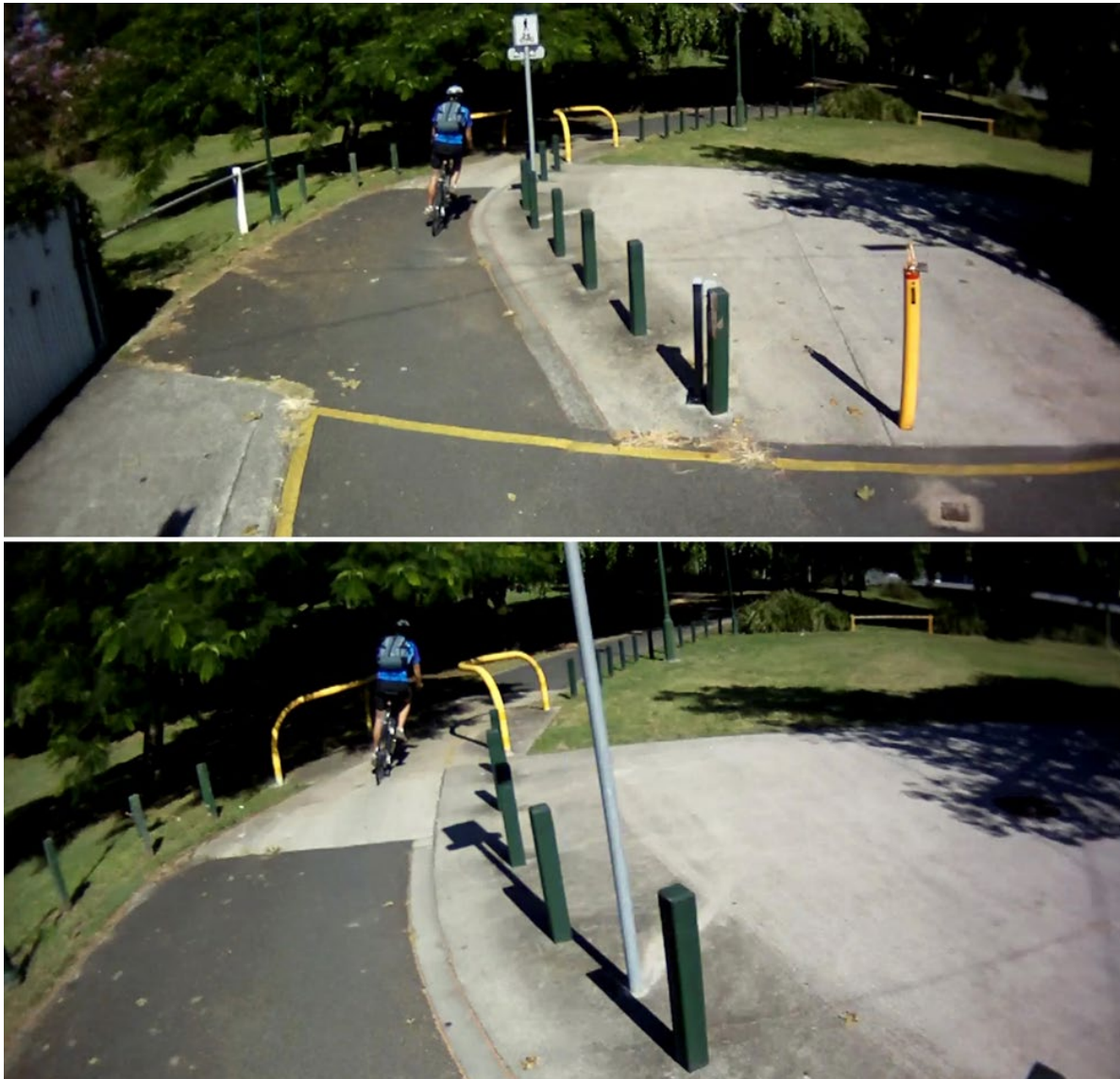
Figure C.21 – Illustration of people riding bikes ‘lean into’ corner turns, and the hazardous positioning of this terminal barrier
