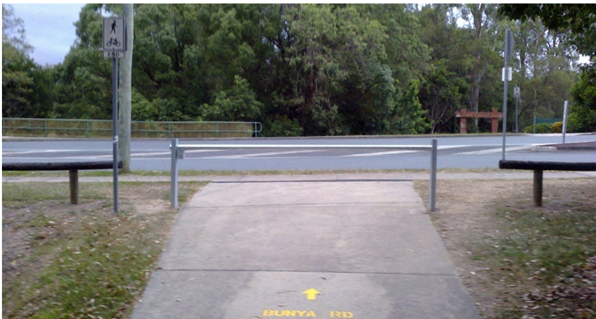
Figure C.8 – Hazardous path terminal device, limited visibility due to lack of contrast
