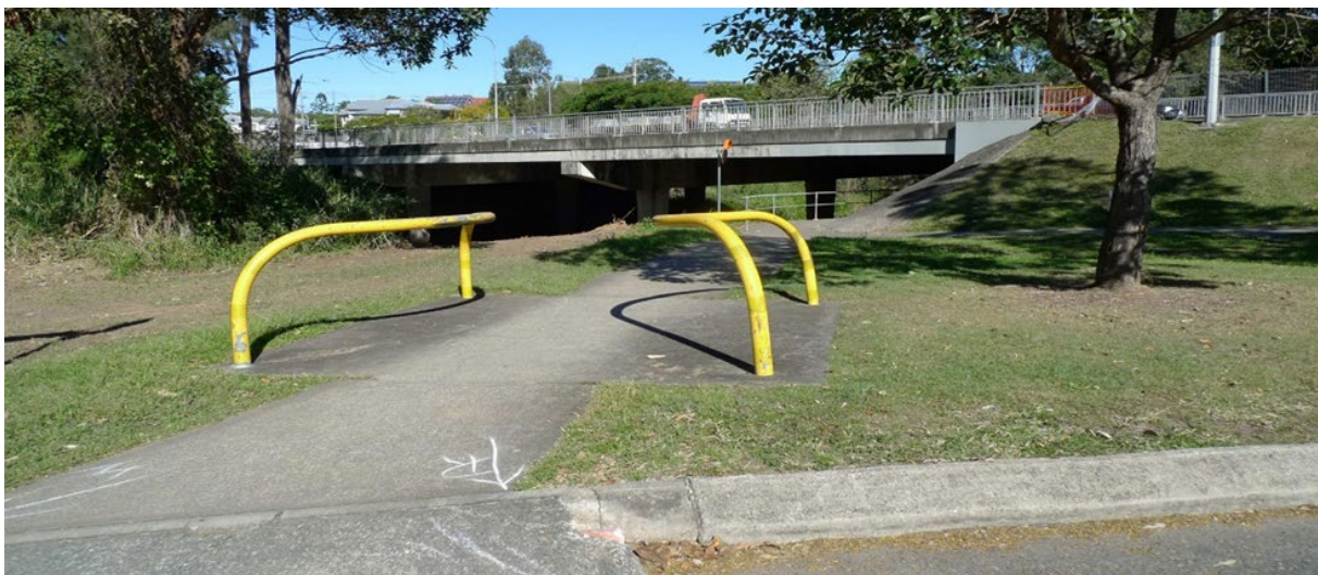
Figure C.3 – Redundant path terminal barrier
