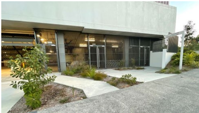
Integrated secured and sheltered bicycle parking facilities at Brisbane South State Secondary College.
