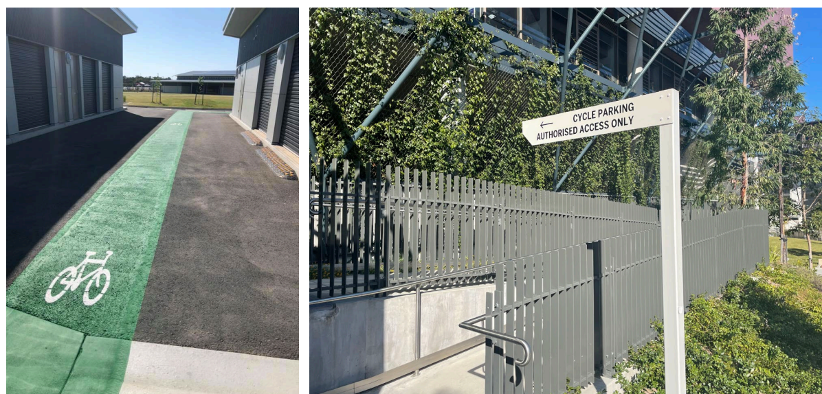
Figure 3.4 – Clear wayfinding signage and line-marking
