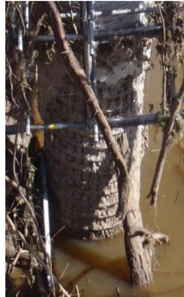
Figure 3.2-3: Unlined piles note the poor connection between the pile and the abutment, particularly on the 3rd and 4th pile
