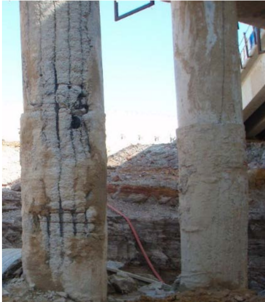
Figure 3.2-3: Unlined piles note the poor connection between the pile and the abutment, particularly on the 3rd and 4th pile
