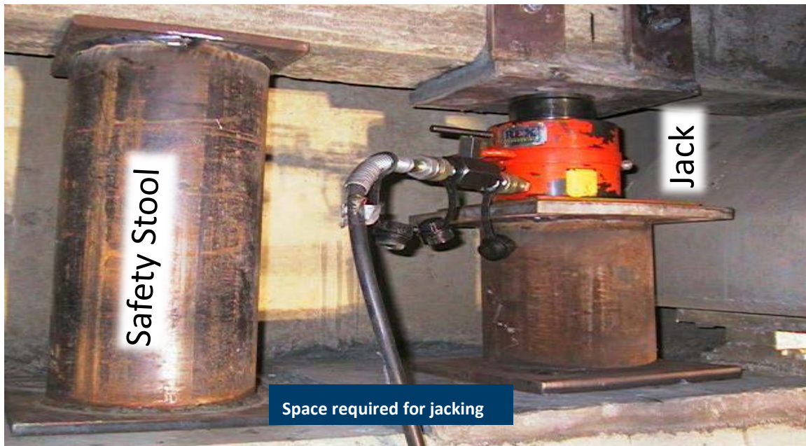
Figure 6.3-2 – Jack and safety stool to support bridge during maintenance work
