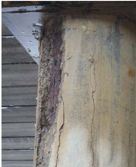
Figure 5.1.2-6: Fallen spall of concrete showing only rust exists where steel reinforcement should be
