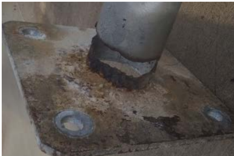
Figure 8.2-2 – Corrosion of buried post
