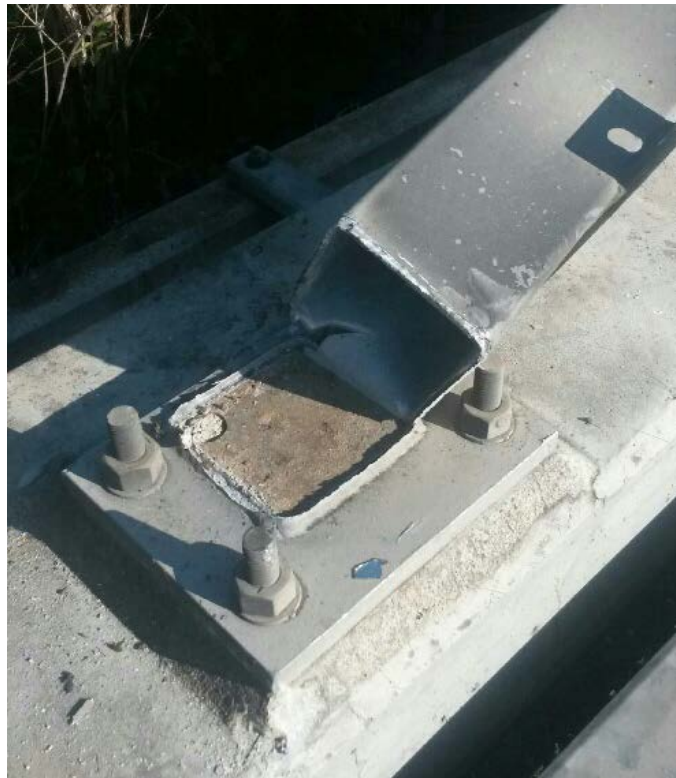
Figure 12-3 – Lack of strength of defective weld
