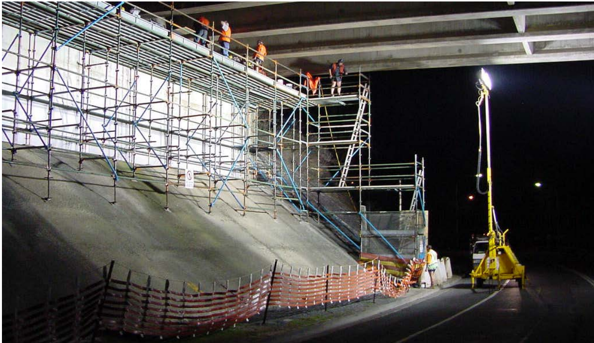
Figure 6.3-1 – Falsework and access for jacking operation
