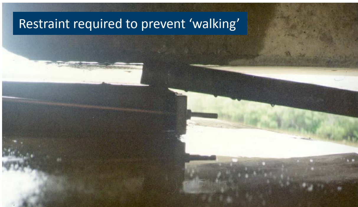
Figure 7.1 – Restraint required to prevent ‘walking’
