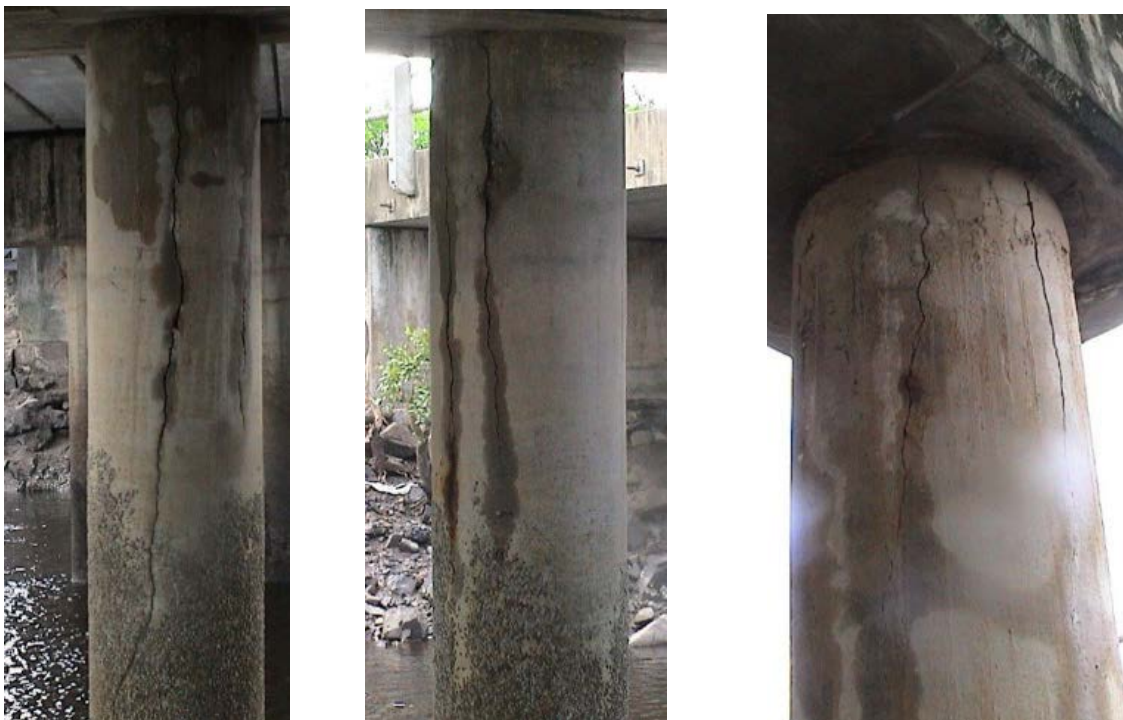
Figure 5.1.2-3: a, b and c: Three hollow spun piles on one project showing typical cracking
