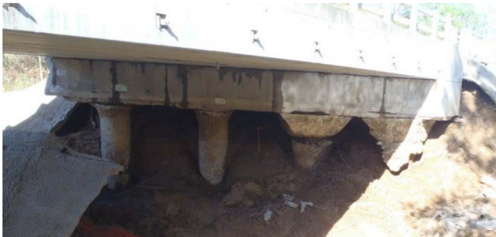
Figure 3.2-3: Unlined piles note the poor connection between the pile and the abutment, particularly on the 3rd and 4th pile
