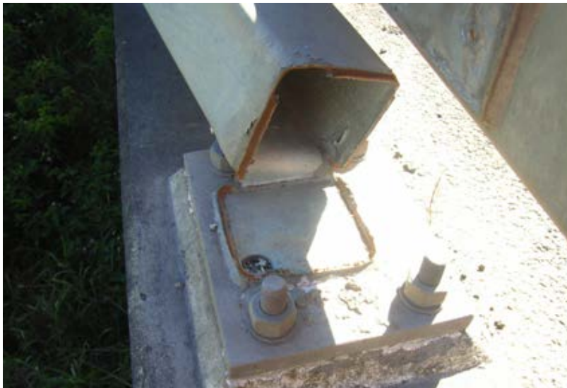
Figure 2 – View of hand rail which failed due to corrosion around the base plate
