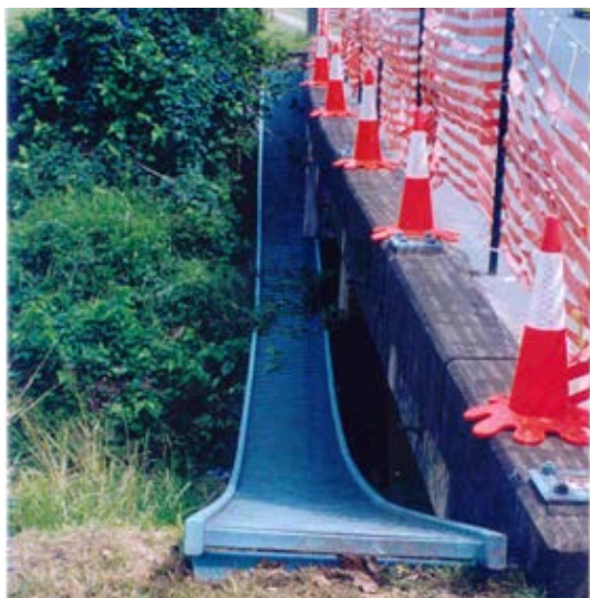
Figure 2 – View of hand rail which failed due to corrosion around the base plate
