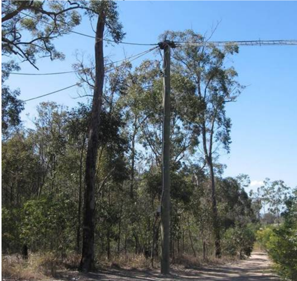
Figure 6.4.3 Canopy bridge at Compton Road, Brisbane. Bridge is connected to the surrounding environment by ropes (Robinson-Wolrath 2007).
