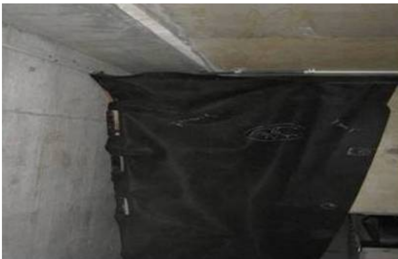
Figure 6.15.2 Blackening screens used to stop any disturbance of areas designated for bat roosting, Brunswick Heads, northern New South Wales.
