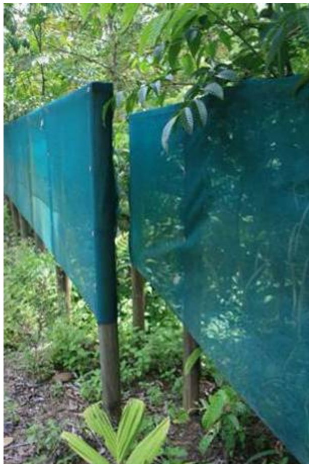
b) Detail of fencing with shade cloth and gap at base
