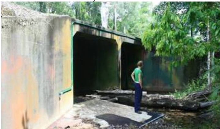
a) Entrance for culvert and showing relative height of passage
