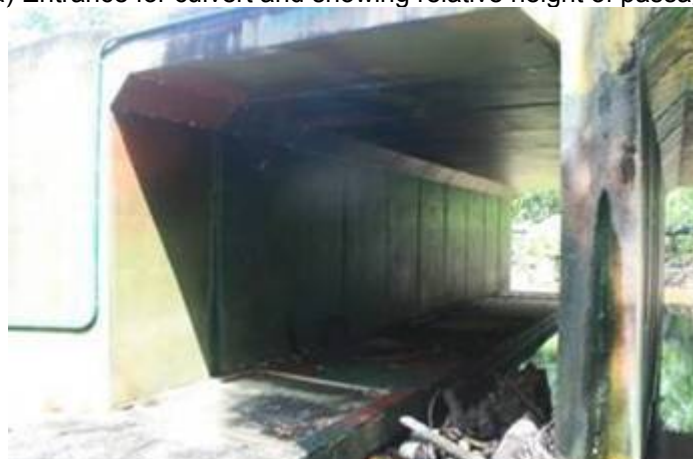
b) Ledge for dry passage within the culvert
