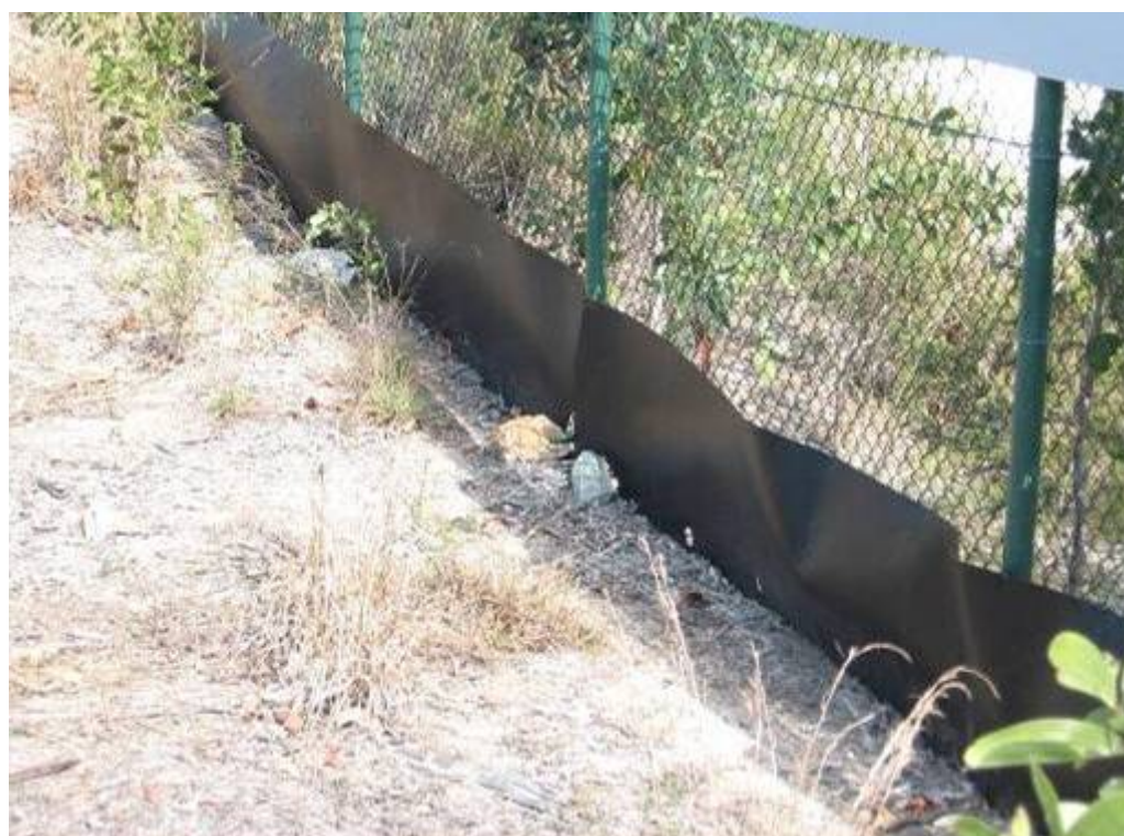
Figure 6.11.5 Fauna exclusion fencing (floppy top) with a three metre clearance buffer on vegetative side, Bonville Upgrade (Roads and Traffic Authority) (Robinson-Wolrath 2007).
