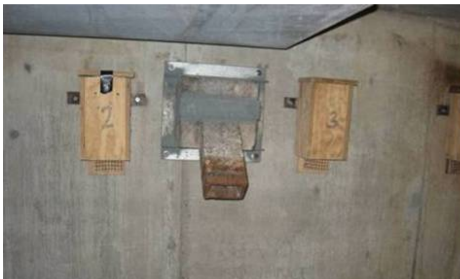
Figure 6.15.3 Timber bat roost under a bridge at Brunswick Heads, northern New South Wales
