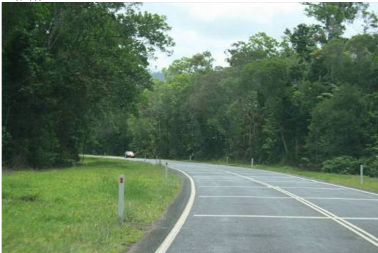
Figure 6.10.5 Rumble strips on the road aimed at slowing traffic in a cassowary area, Mission Beach, Queensland.
