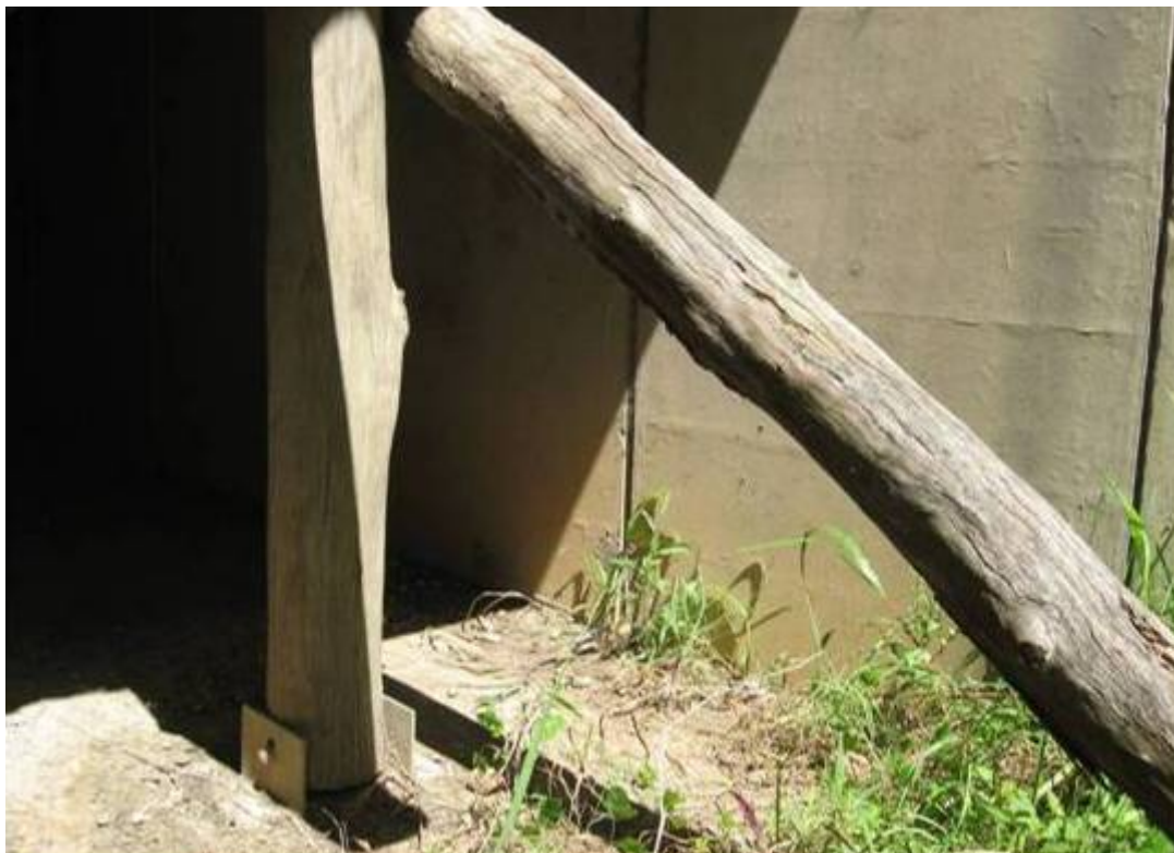
Figure 6.6.13 Lead up pole to a horizontal log used to traverse the culvert at a safe height (Robinson-Wolrath 2008).
