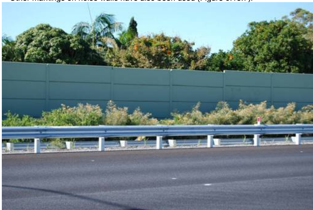
Figure 6.18.6 Solid noise wall barrier (Taylor 2008).
