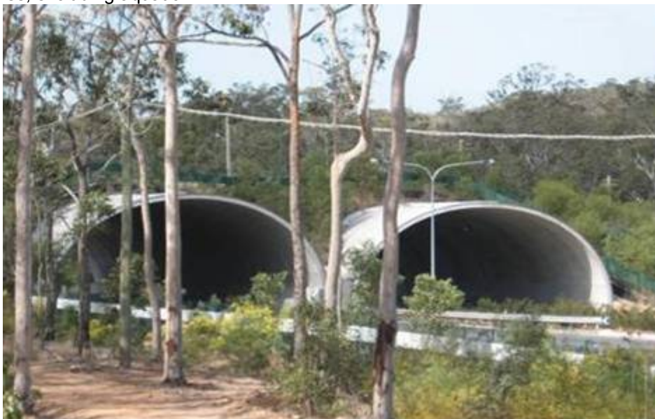
Figure 6.1.1 Land bridge at Compton Road, Brisbane (Robinson-Wolrath 2007). Rope ladder installed to cater for arboreal species.
