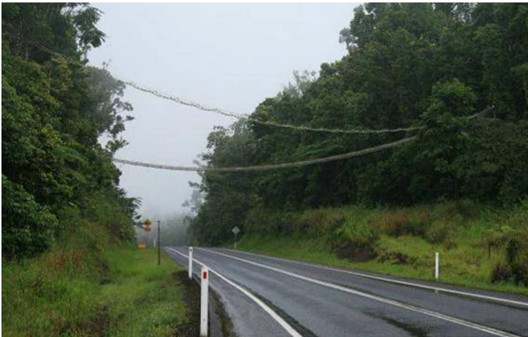
Figure 6.4.1 Canopy bridges (ladder and box) over Palmerston Highway, North Queensland (Scott 2007).
