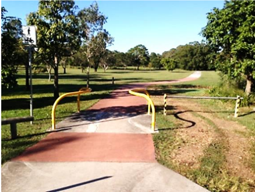
Figure 2.4.1.3 – Maintaining vehicle access in facility management
