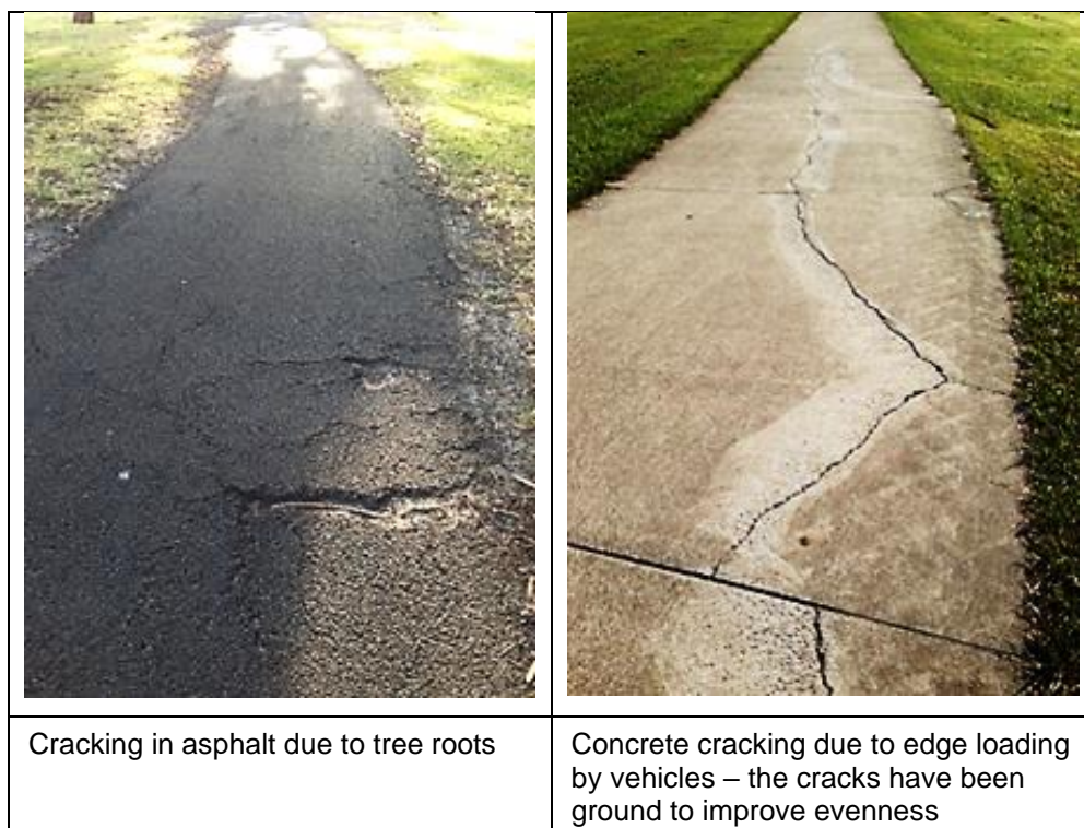
Figure 2.1.5.3 – Maintenance of cracking in pathway pavement
