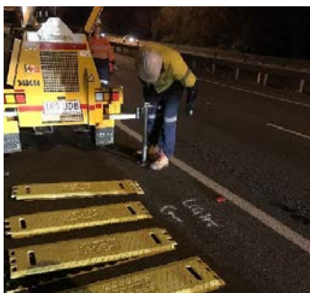
Workers install Road Quake rumble strips on suitable roadworks sites on the Gateway Motorway. This type of rumble strip is beneficial because it is temporary, portable and durable.
