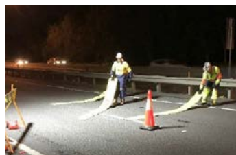
Workers install Road Quake rumble strips on suitable roadworks sites on the Gateway Motorway. This type of rumble strip is beneficial because it is temporary, portable and durable.
