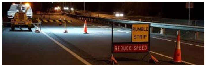
Workers install Road Quake rumble strips on suitable roadworks sites on the Gateway Motorway. This type of rumble strip is beneficial because it is temporary, portable and durable.
