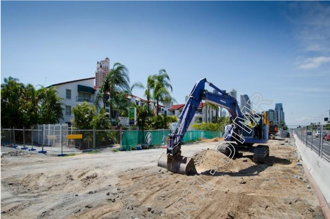
Figure 3: Pavement Preparation works in front of Mardi Gras
