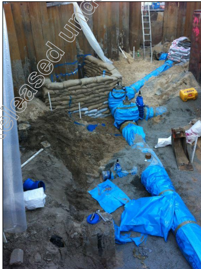
Figure 11: Thrust Block Preparation of W7 at Wharf Rd
