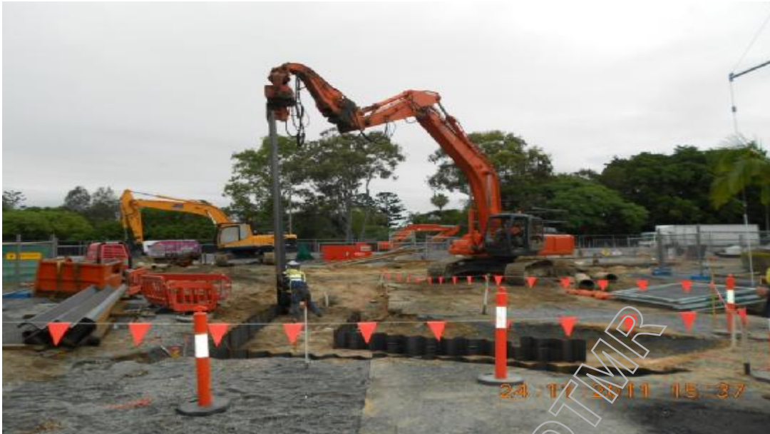
Figure 5: Sheetpiling in Progress at the S11 Sewer
