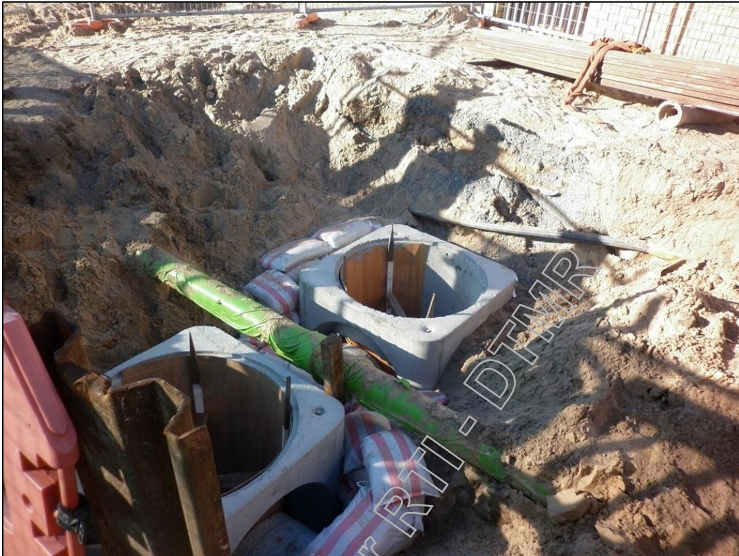
Figure 14: Precast Stormwater Pits
