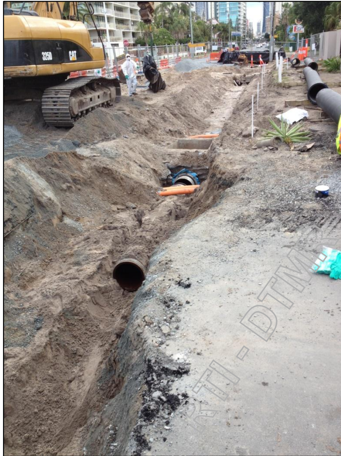
Figure 8: DN375 Installation Nth of Aubrey
