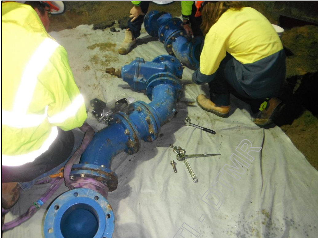
Figure 4: Assembly of the W3 Watermain Nth of Fern
