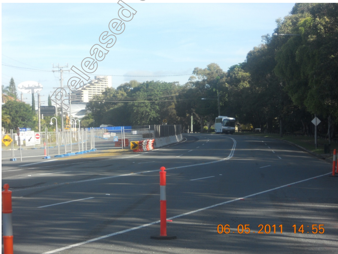
Completed Southern Stage 2 Traffic Switch
