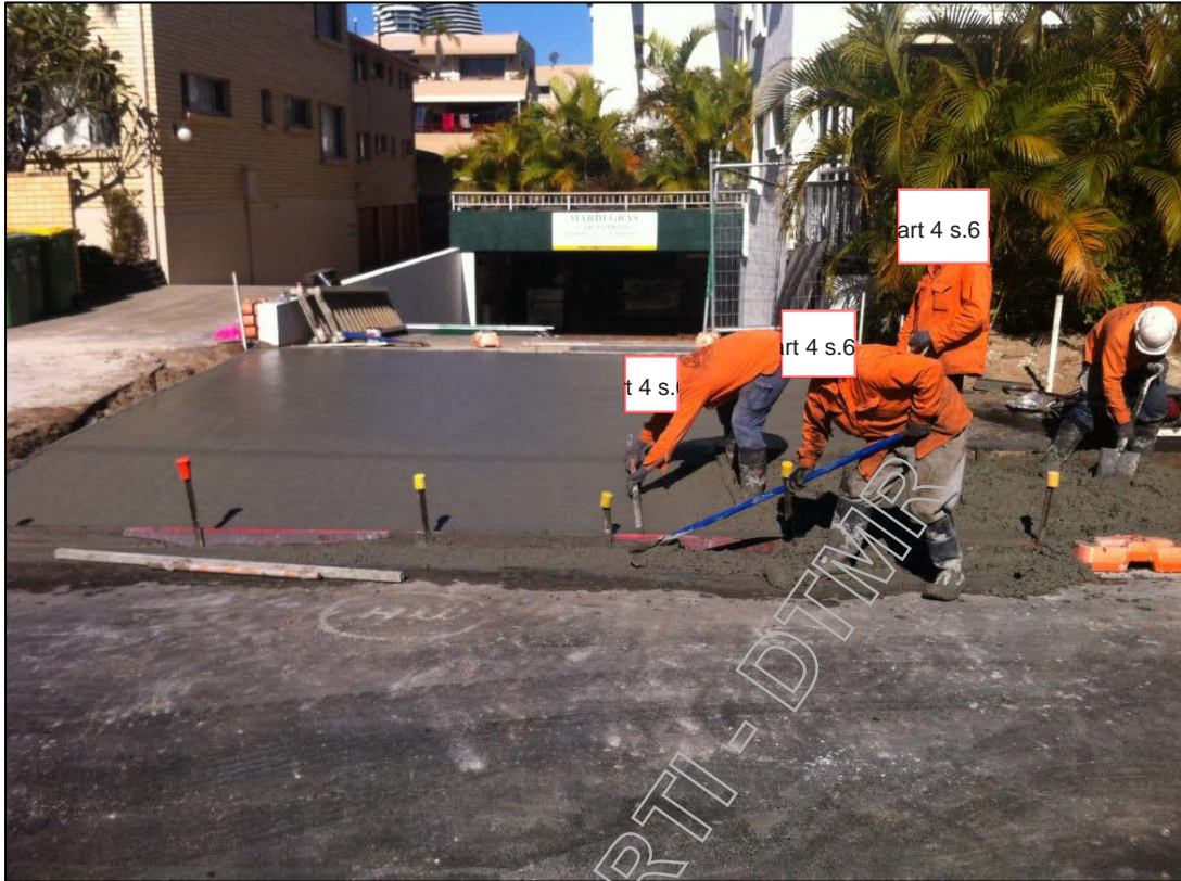
Figure 16: Pouring of Mardi Gras Driveway
