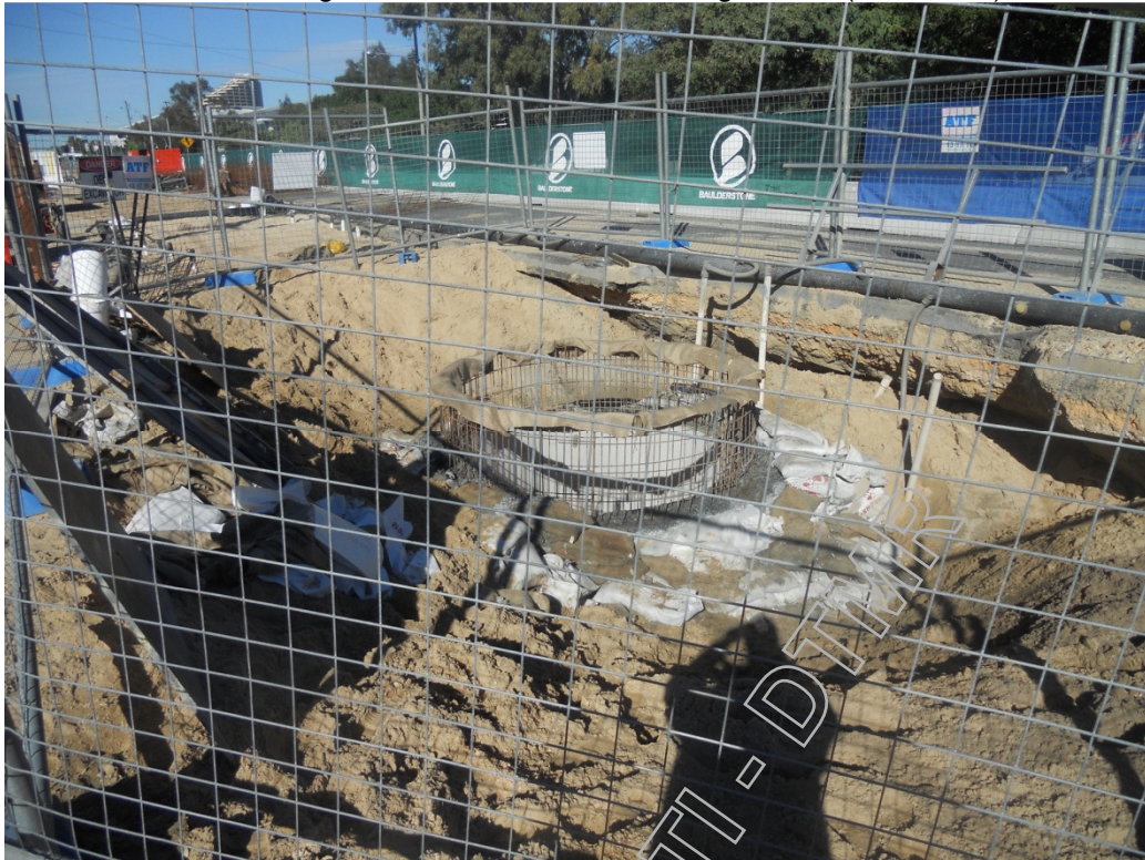
Southern Stage 2 – Stormwater drainage manhole construction
