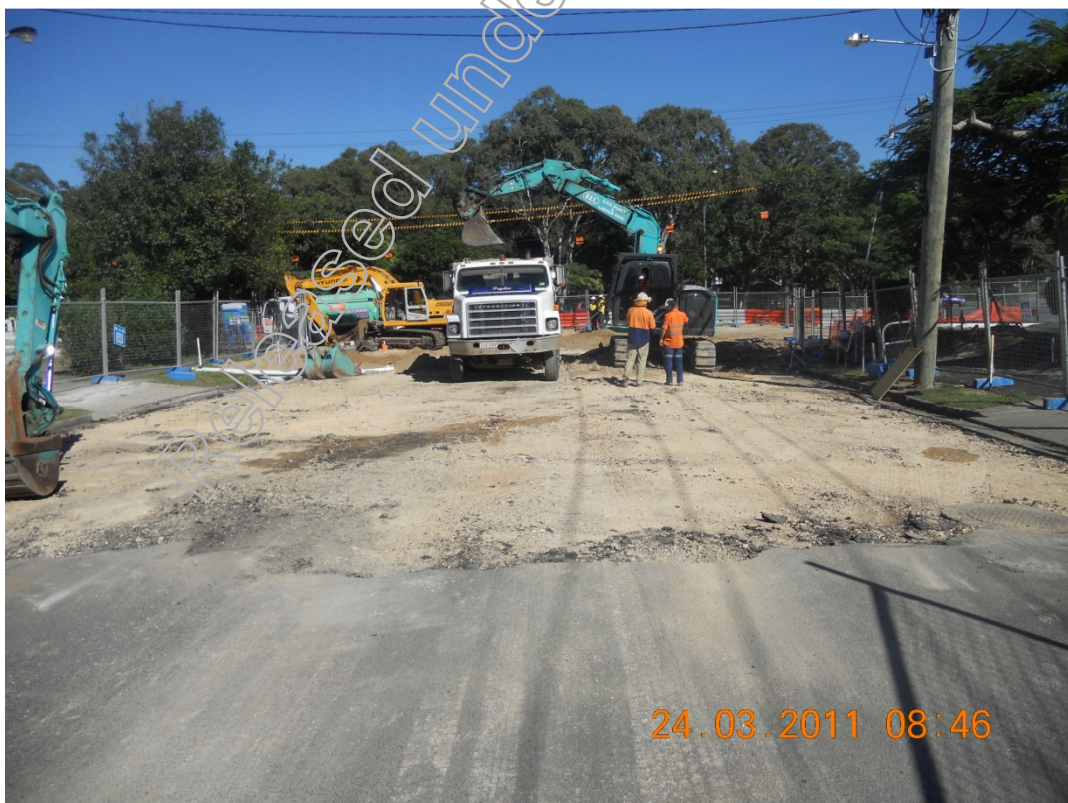
Pavement construction in Armrick Ave
