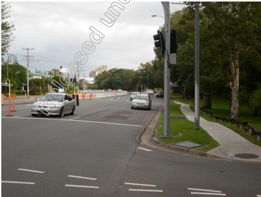
Southern Stage 2 traffic switch preliminary works
