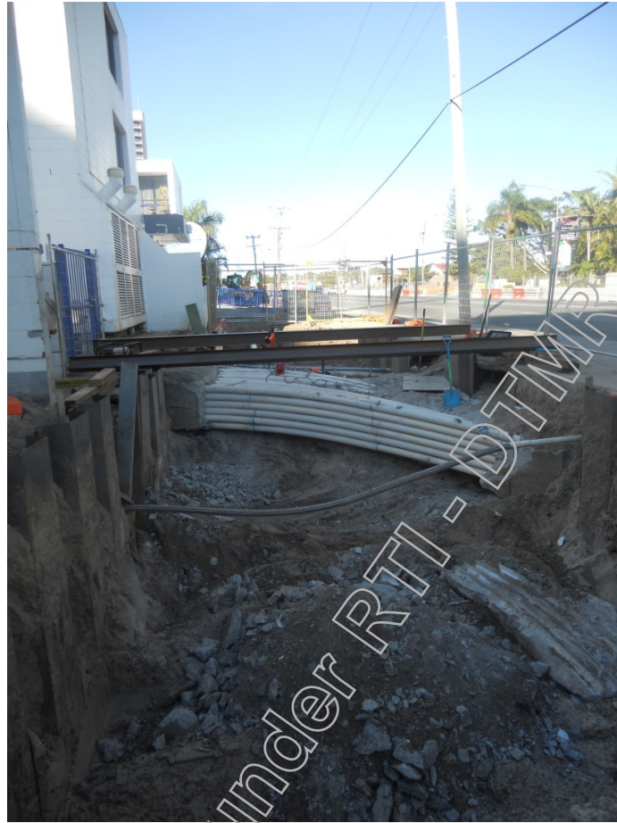
Manhole 89 – Sheet piles installed and removal of concrete encasement of Telstra network commenced
