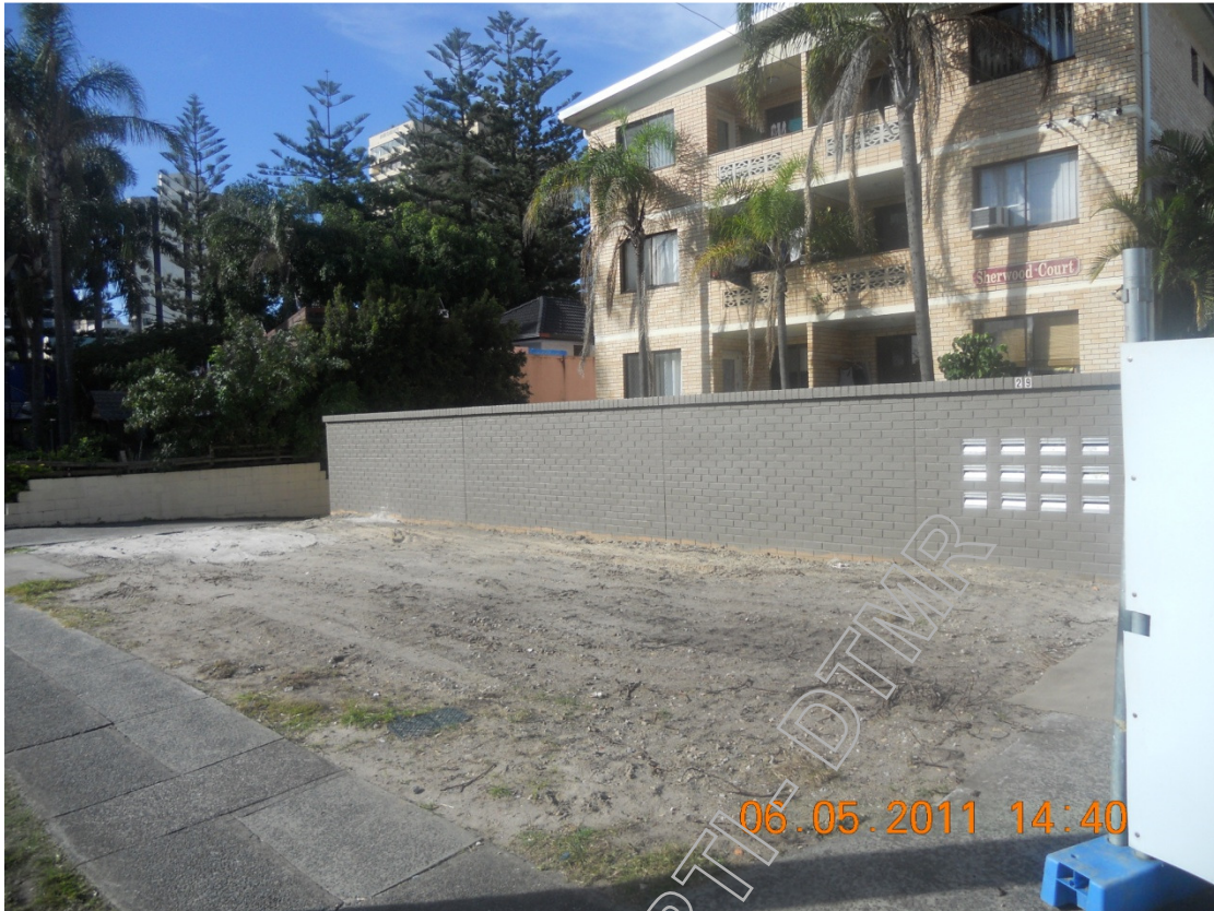
Completed Property Accommodation works – Sherwood Court
