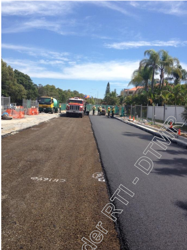
Figure 7: Asphalt and Curb Progress North of Australia Avenue (Mid Feb)
