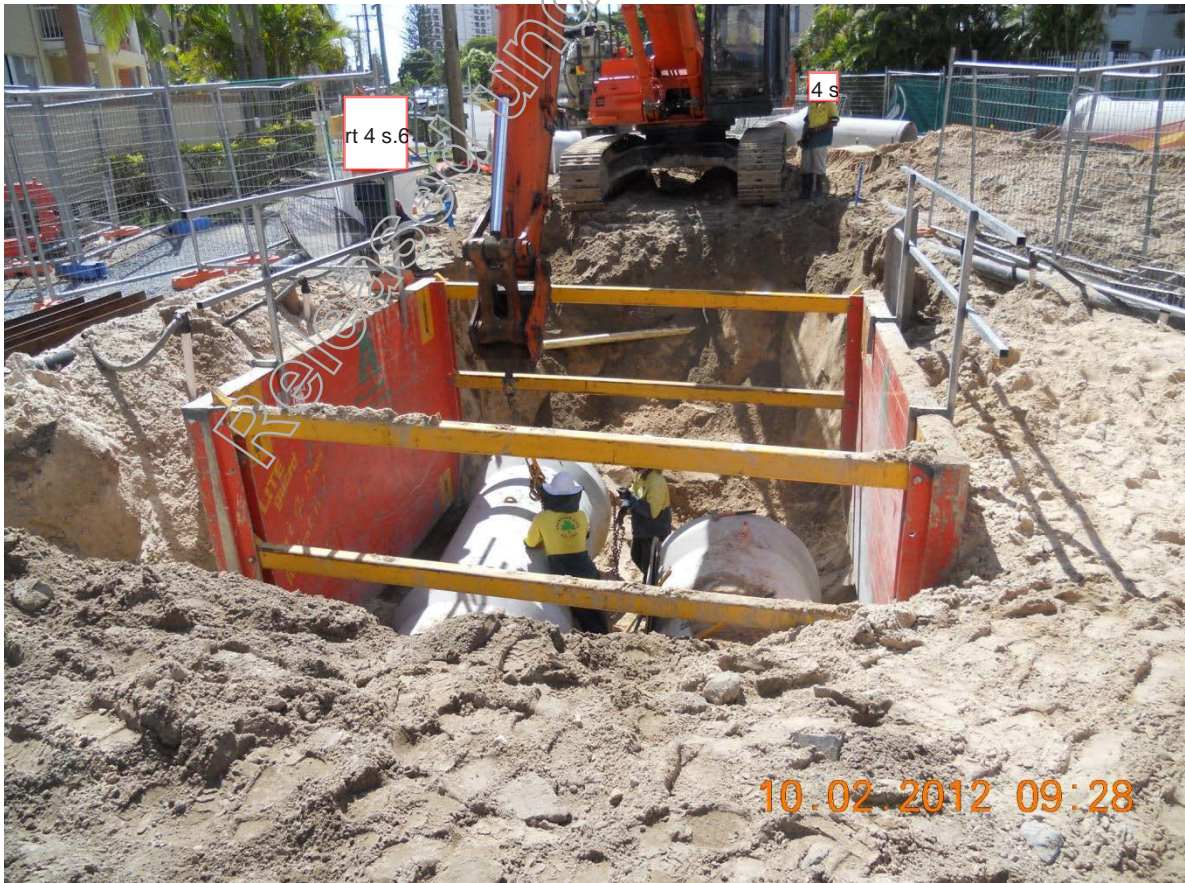
Figure 6: Twin 1200Ø Stormwater Drainage Pipes of Section 3/9 at Britannia Av
