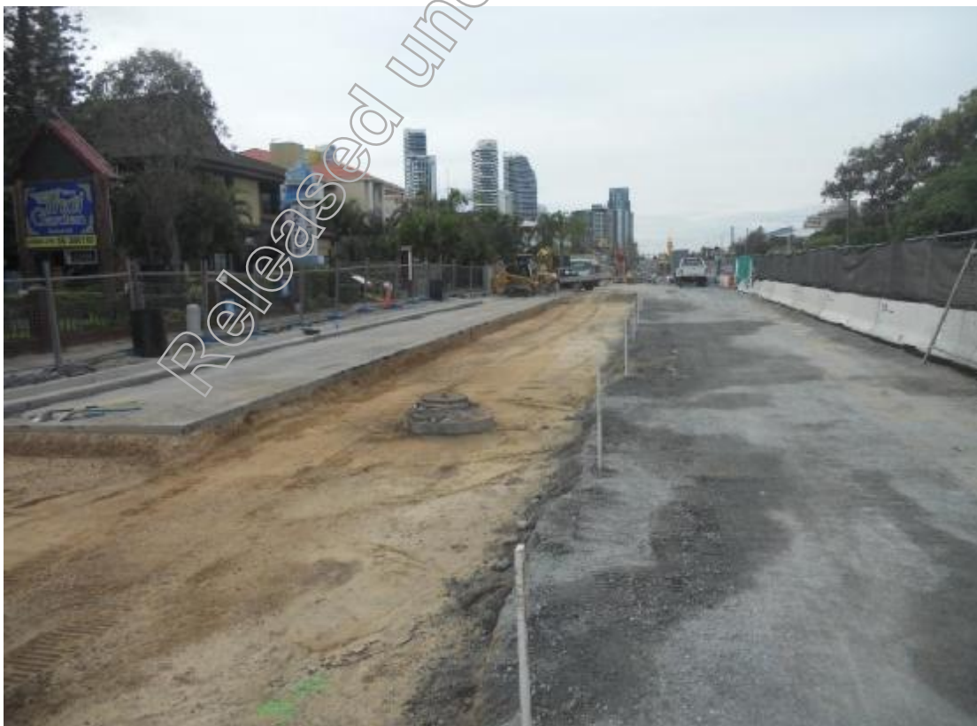
Figure 2: Pavement preparation works at Chelsea Avenue (to be open for Christmas)
