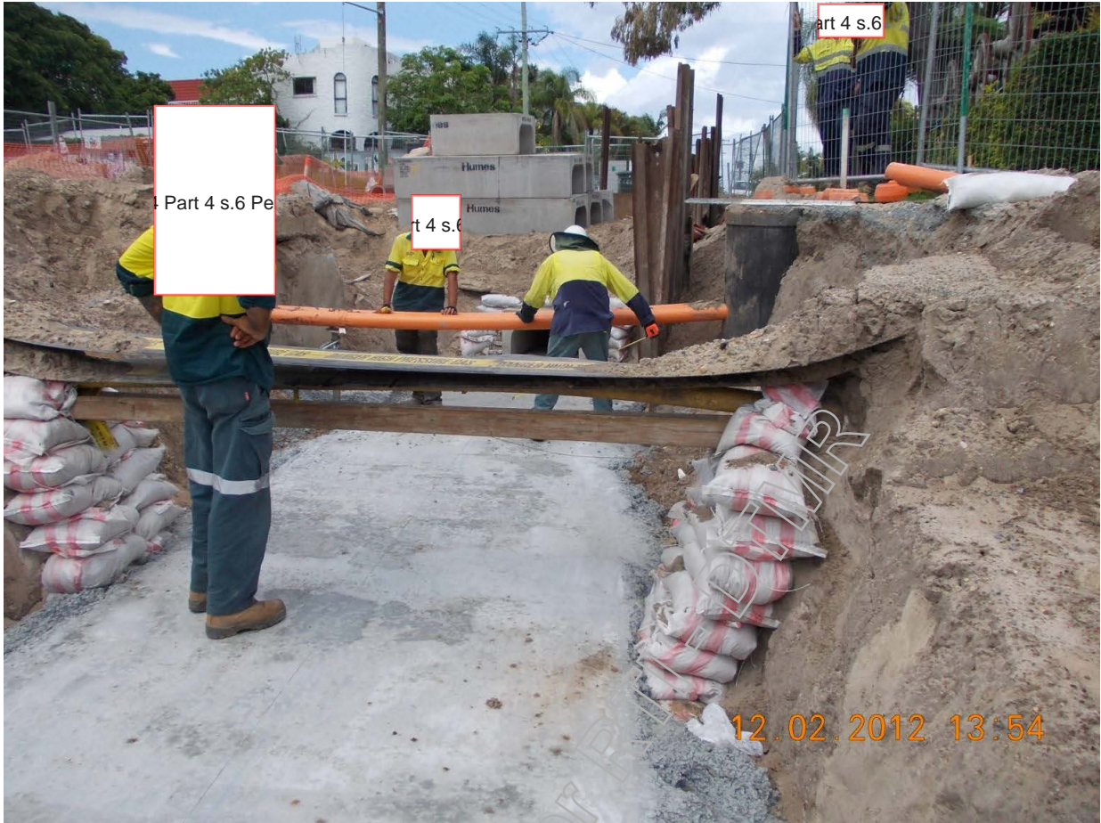
Figure 5: 750x375 Box Culvert Installation of 1/14 and 2/14 at St. Kilda Avenue
