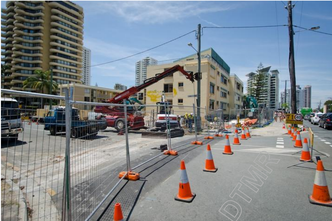
Figure 7: Energex works at Aubrey St
