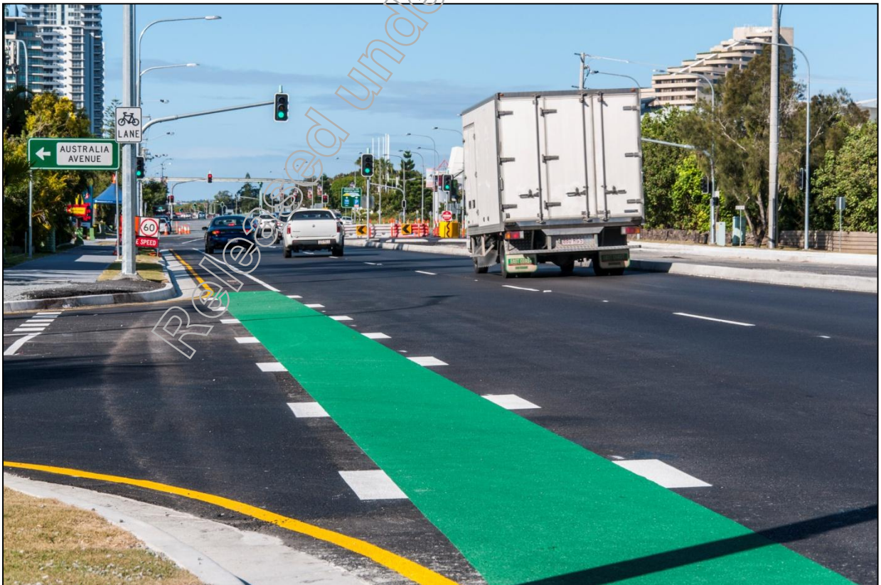
Figure 3: New Kerb, Pavements and Line Marking near Britannia Av
