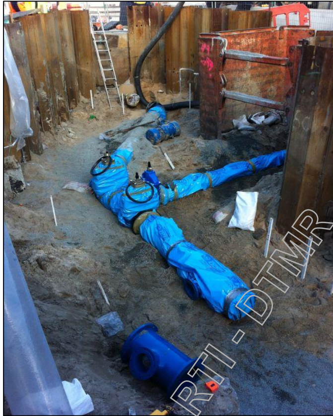
Figure 10: W7 Installation At Wharf Rd
