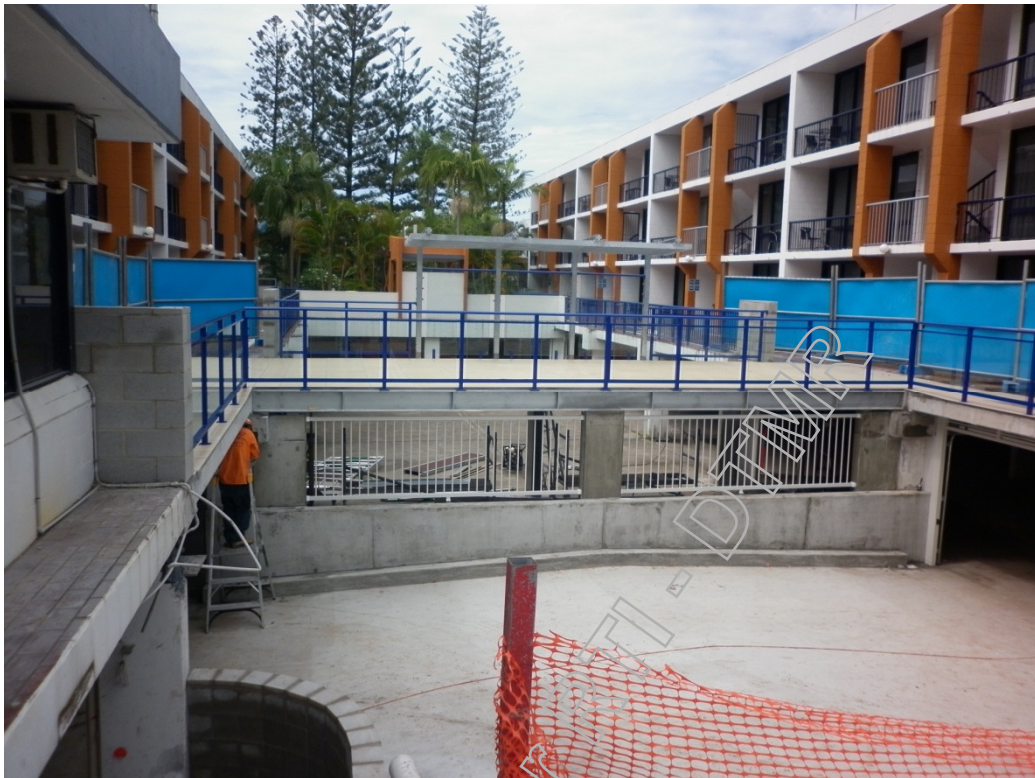
Club Surfers Property Adjustment works – Near completion
