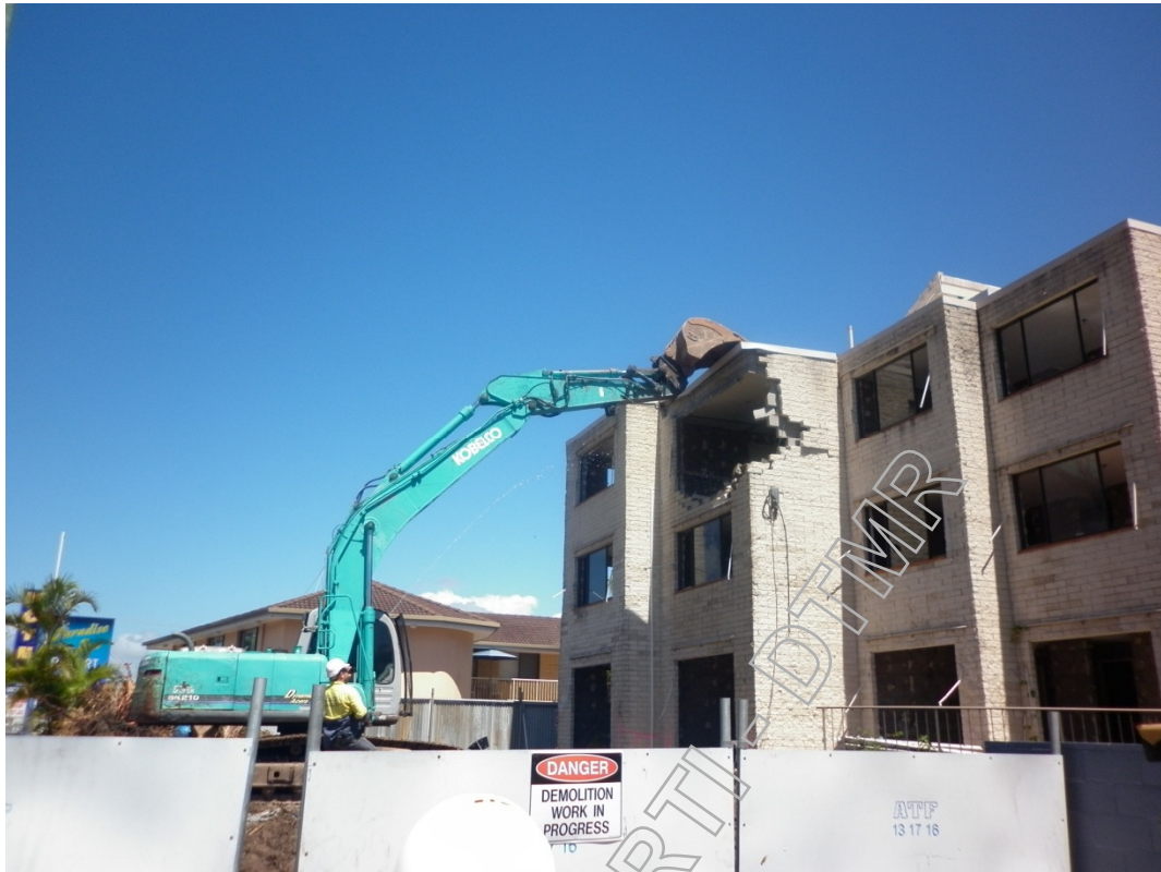
Commencement of St Moritz Mechanical Demolition
