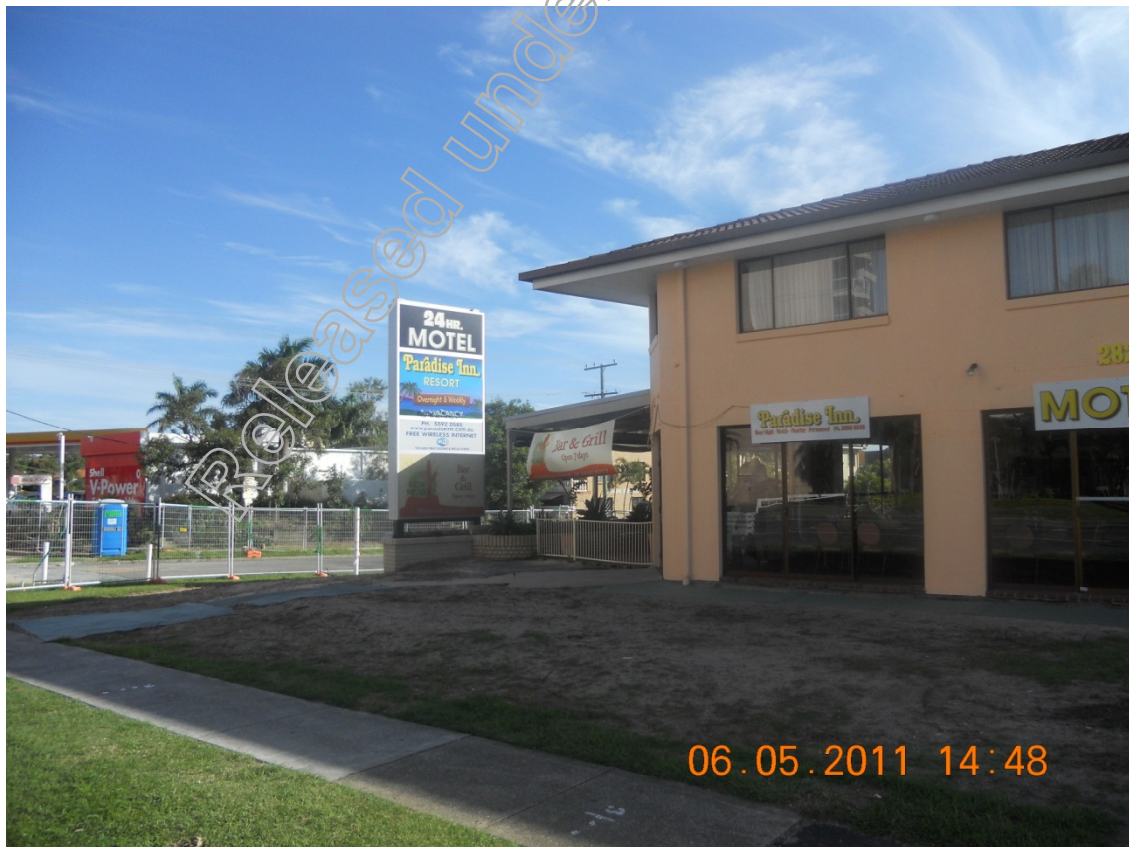
Completed Property Accommodation works – New Mexico/Paradise Inn
