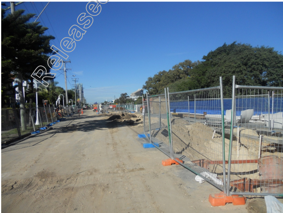
Manhole 89 – Sheet piles installed and removal of concrete encasement of Telstra network commenced
