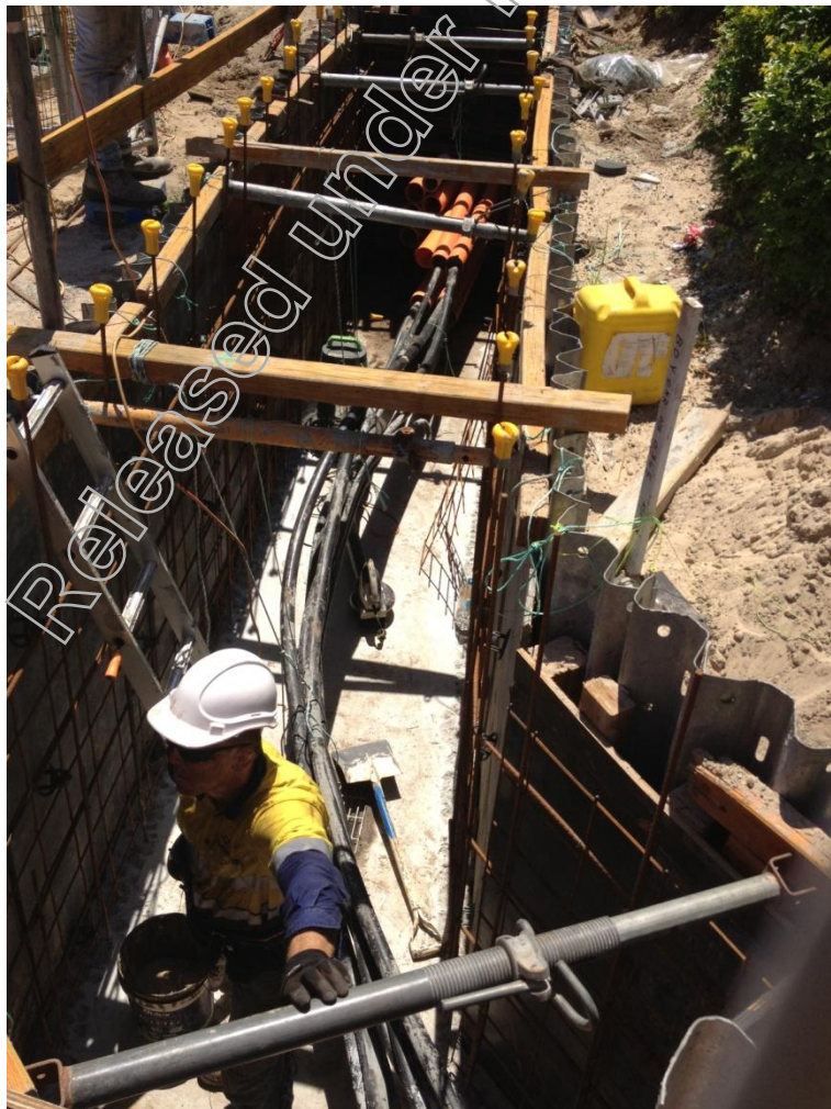
Figure 4: Electrical Pit 50 Installation at St. Kilda Avenue
