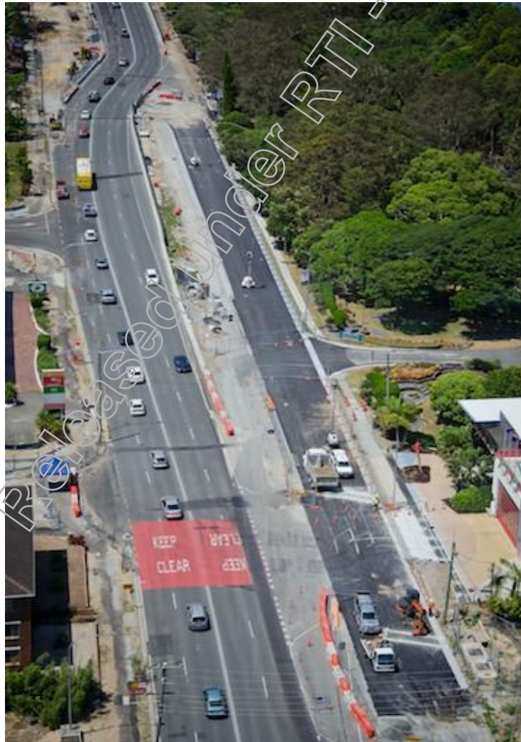
Figure 6: Completed Asphalt works at Cascade Gardens
