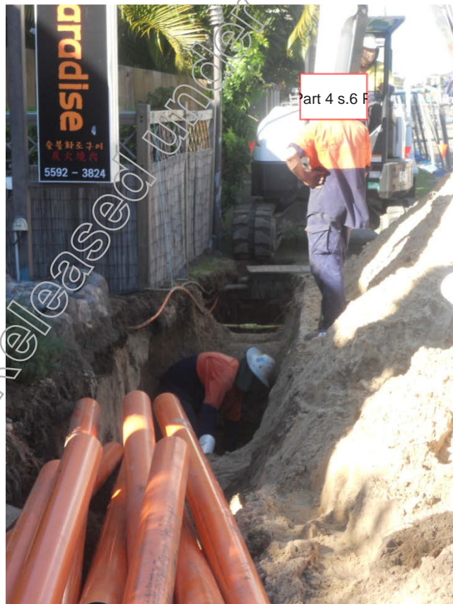
Southern Stage 2 – Installation of Energen network in close proximity to properties
