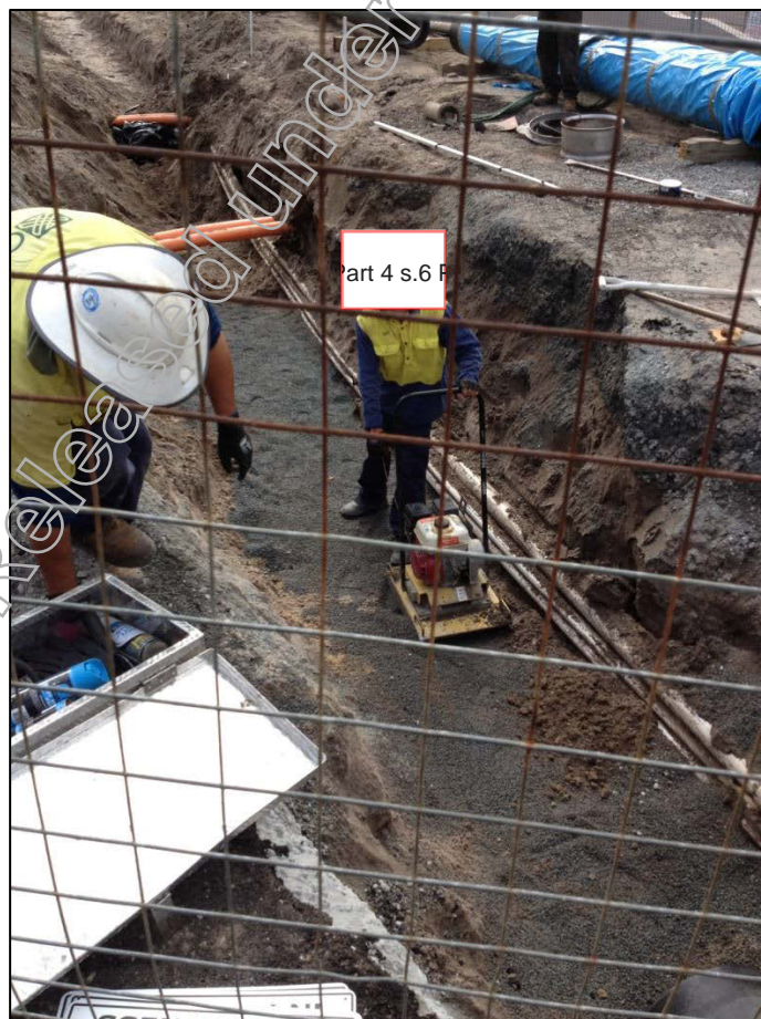
Figure 7: Backfill of the DN375 AC to DICL Nth of Frederick
