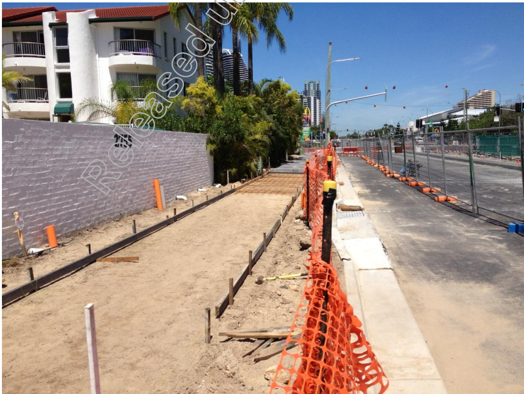
Figure 8: Asphalt Completion and Pavement Works North of Australia Avenue (Late Feb)
