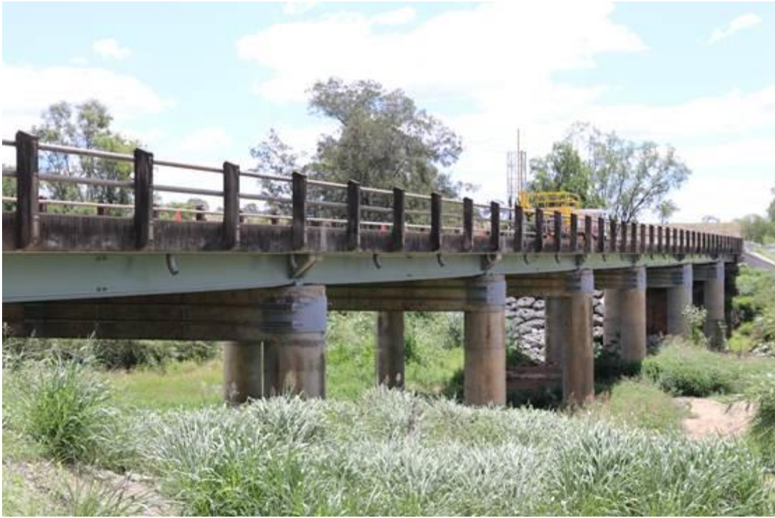
Rehabilitation and strengthening works on the Lockyer Creek Bridge
