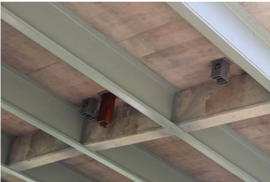
Two types of bat boxes on the underside of Lockyer Creek Bridge to encourage micro-bats to return after the completion of rehabilitation and strengthening works
