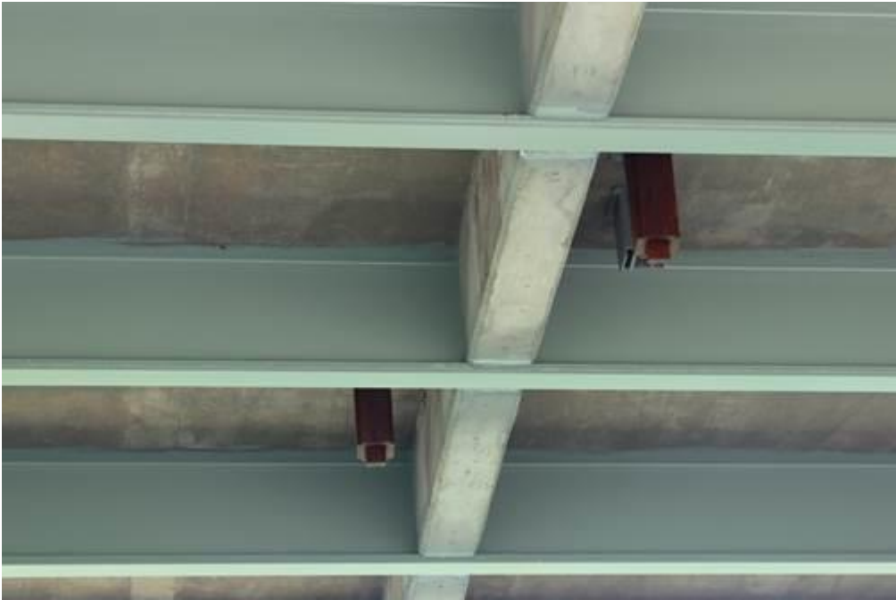
Two types of bat boxes on the underside of Lockyer Creek Bridge to encourage micro-bats to return after the completion of rehabilitation and strengthening works
